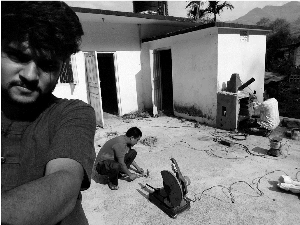
Plate 3 Plant under construction (metal works)
