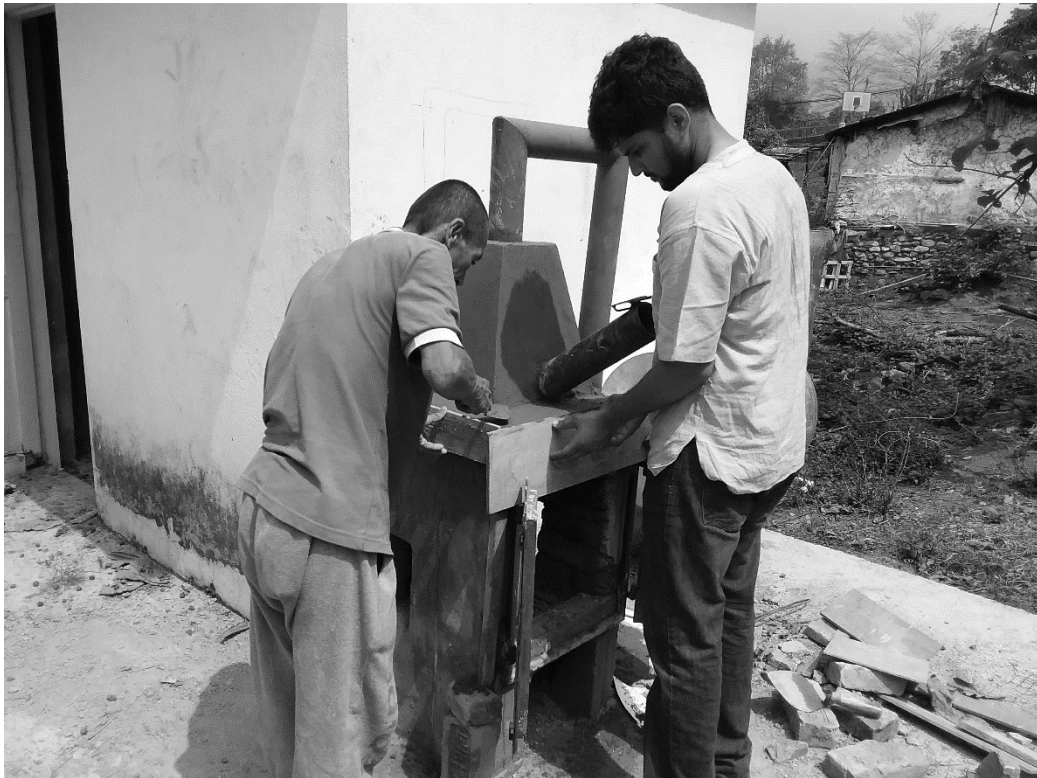
Plate 4 Smoke generation chamber under construction
