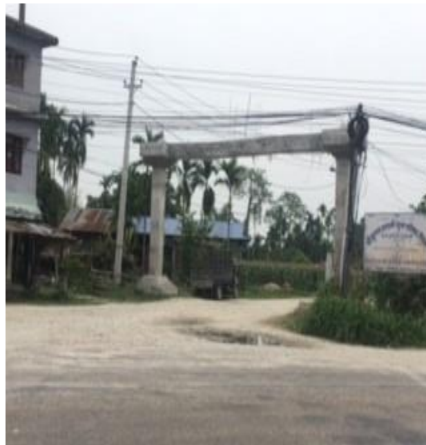
c) Pranami Nagar entrance
